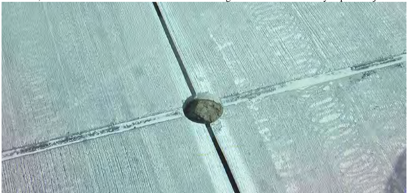
Fig. 2. Crossing Concrete Pad Expansion Joints with The LEDline® Direct Burial Power Line:
